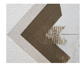
Drying type compounds will shrink and harden with evaporation of water. The joints must be allowed to set and appear completely dry before re-coating or sanding. Actual drying times will be extended in low temperature and high humidity conditions. Do not use a setting type compound over a drying type compound.
